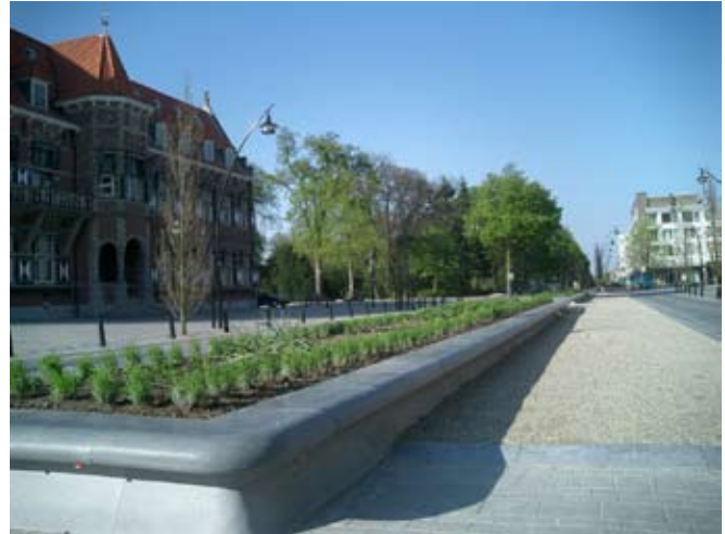
beplanting in meubelairstrook
