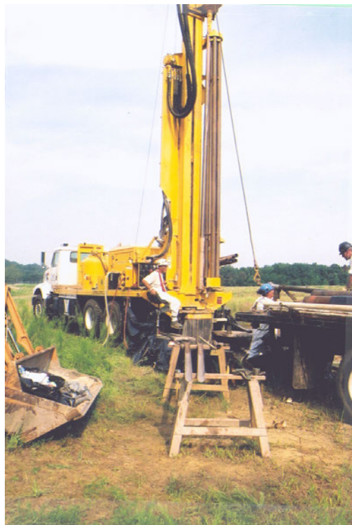
An air rotary drilling rig installing a new groundwater monitoring well at the Letart Landfill.
